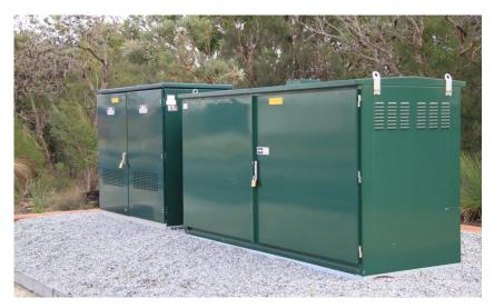
Figure 57: HV outdoor ground mounted switchgear & transformer
