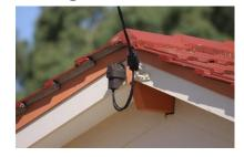
Figure 14: Standard overhead connection and PoA
