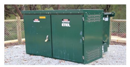
Figure 55: Modular package substation
