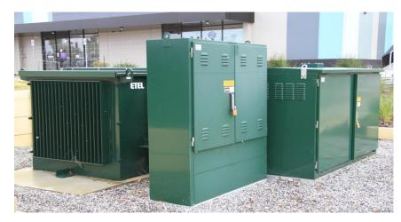
Figure 56: Non modular package (cluster) substation arrangement
