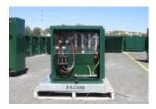
Figure 13: Rural/SPUD transformer supply (1 phase)
