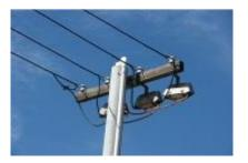
**Figure 17:** Commercial 3 phase 4 single core connection
