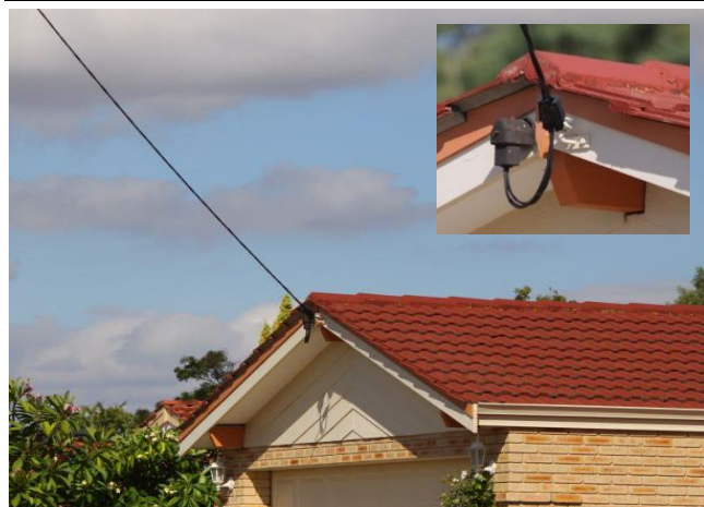
Figure 2: Larger than standard supply - overhead three-phase (bare)
