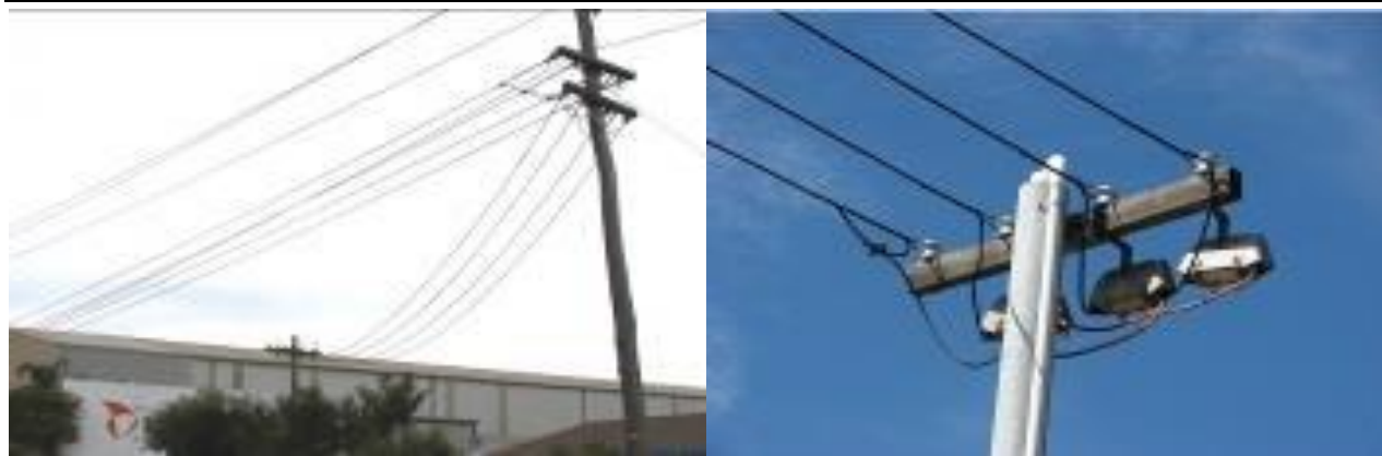
Figure 2: Larger than standard supply - overhead three-phase (bare)
