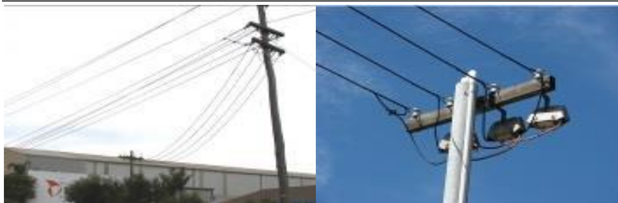
Figure 2: Larger than standard supply - overhead three-phase (bare)
