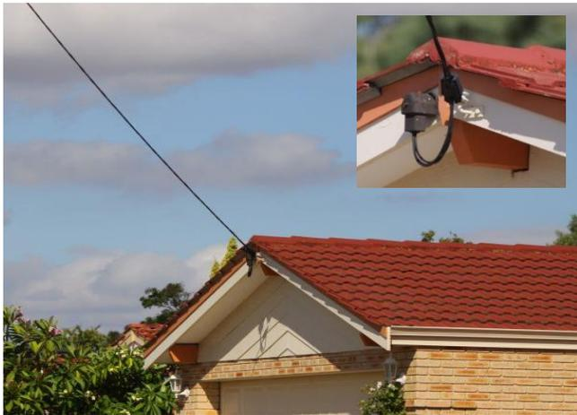
**Figure 2: Larger than standard supply - overhead three-phase (bare)**
