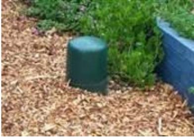
Universal pillars (commonly referred to as uni pillars) have the same appearance as mini pillars but they are slightly bigger at 480 mm diameter. In residential areas, uni pillars are used for switching point in the LV network but can also provide standard supplies to residential premises. Commercial and industrial premises are commonly supplied with a dedicated uni pillar to provide a larger than standard supply on a shared LV feeder.
