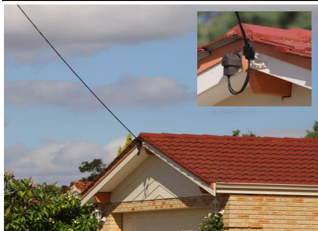
Figure 2: Larger than standard supply - overhead three-phase (bare)
