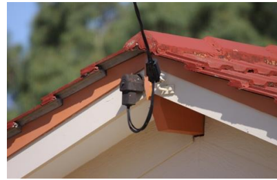
Figure 14: Standard overhead connection and PoA
