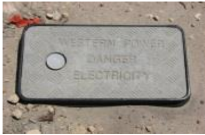
Figure 8: Below ground UMS pit
