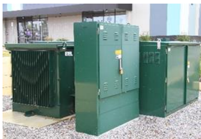
Figure 12: Non MPS (cluster) substation
