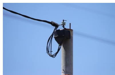
Figure 15: Domestic aerial service cable connection (3 phase)
