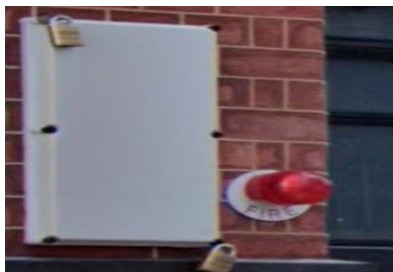
Figure 10: 100A/200A cut out box
