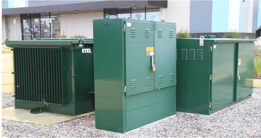
Figure 56: Non modular package (cluster) substation arrangement
