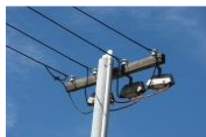
Figure 17: Commercial 3 phase 4 single core connection
