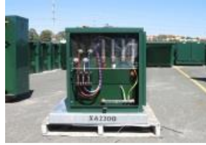
Figure 13: Rural/SPUD transformer supply (1 phase)
