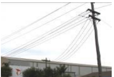
Figure 17: Commercial 3 phase 4 single core connection
