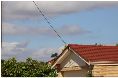
Figure 14: Standard overhead connection and PoA
